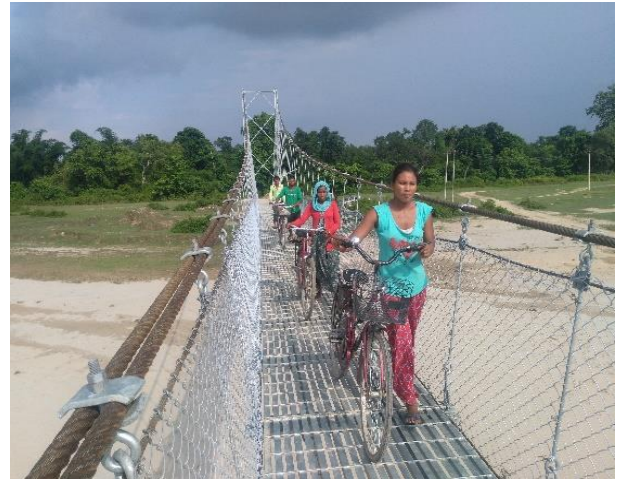
Women crossing the Pattharbojhi trail bridge safely and easily after the construction of the trail bridge
